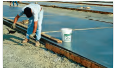
Step - 3 Strip form and insert dowel into SPEED DOWEL ®
