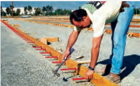
Step - 1 Attach base to edge form and tap on sleeve
